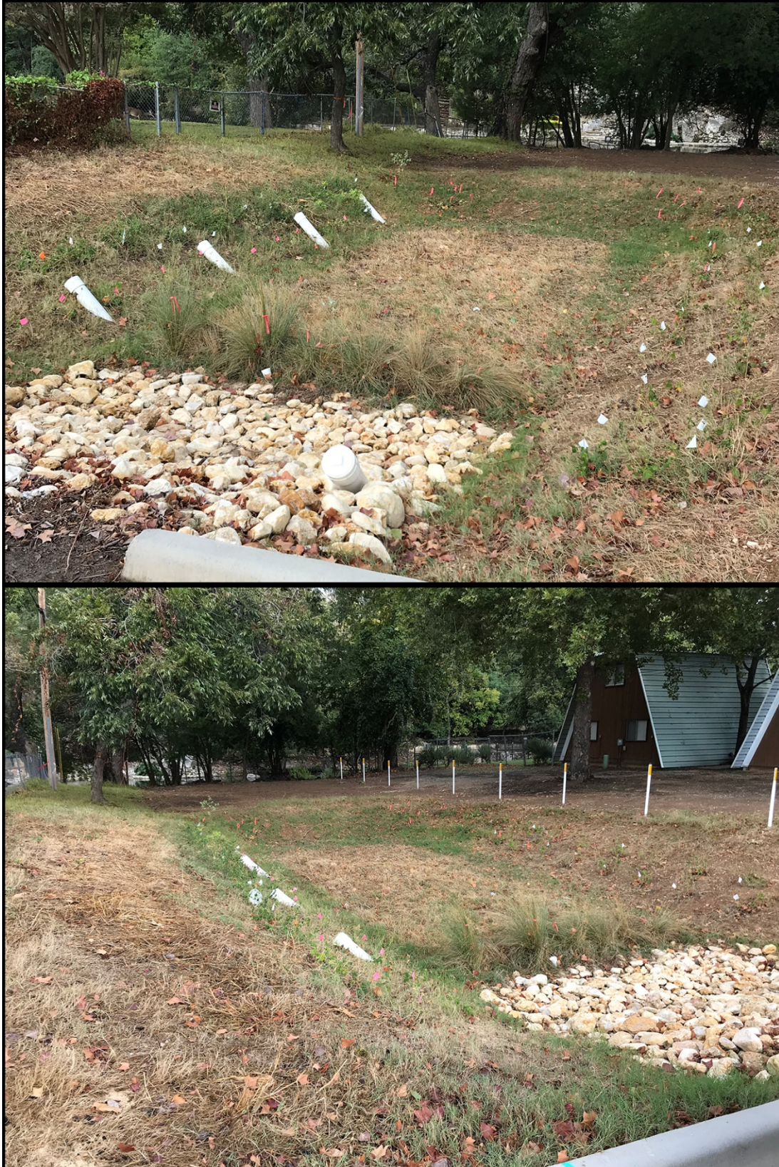
Figure 6.2-14. Photos showing bio-retention basin constructed at North Houston Avenue adjacent to Upper Spring Run of Landa Lake.
