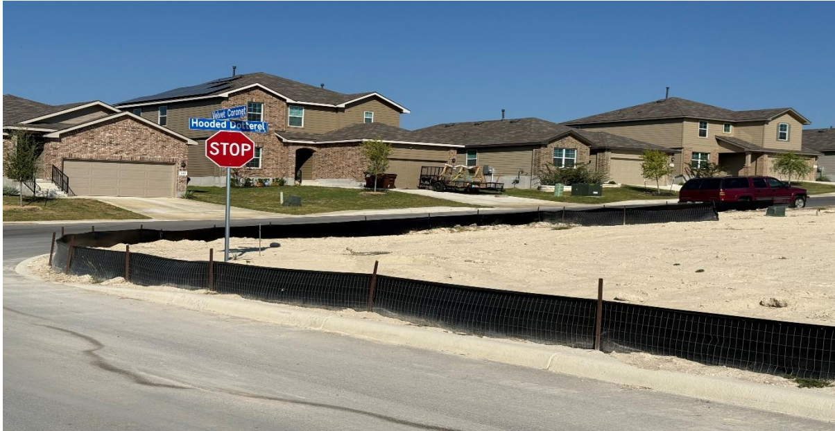
Exhibit F: Road Construction and Silt Fencing
