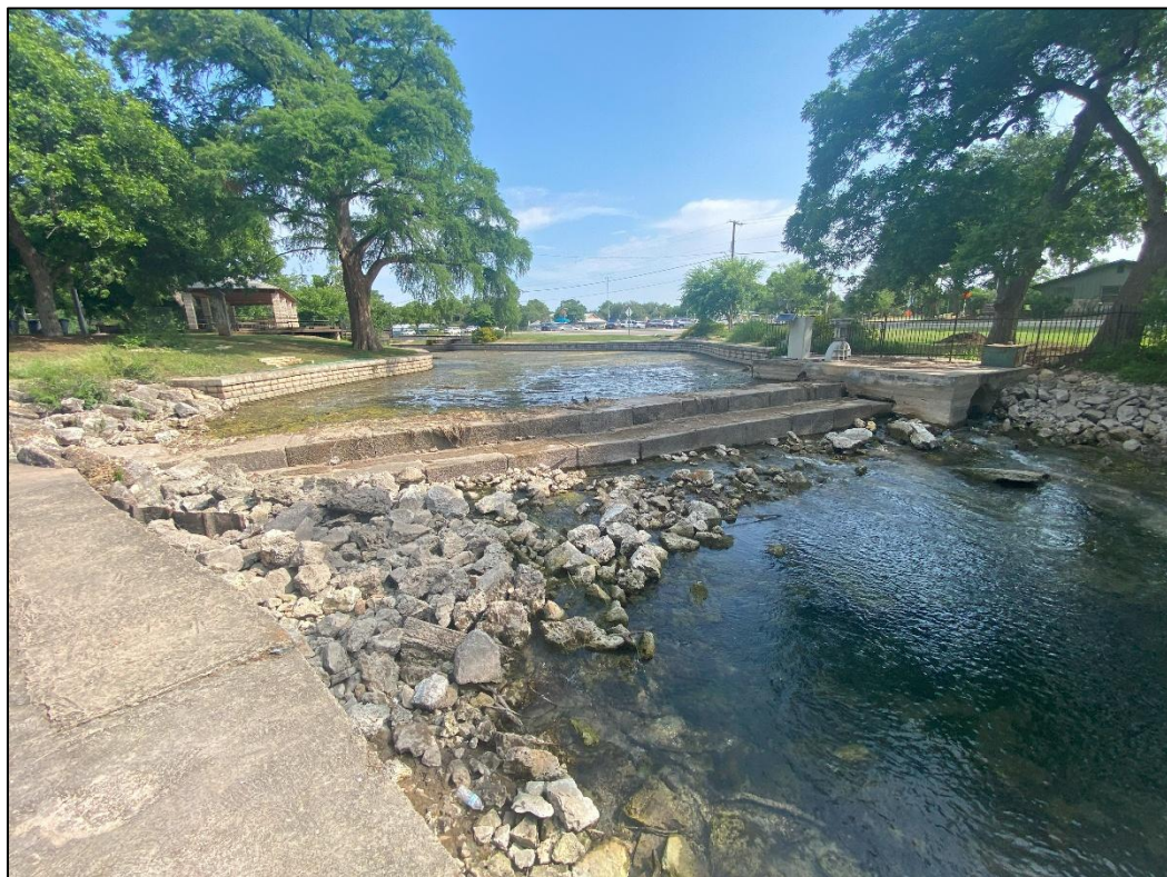
Figure 23. Weir dam holding water in the New Channel at 50 cfs. Water was still flowing through the culvert (May 21 st ).
