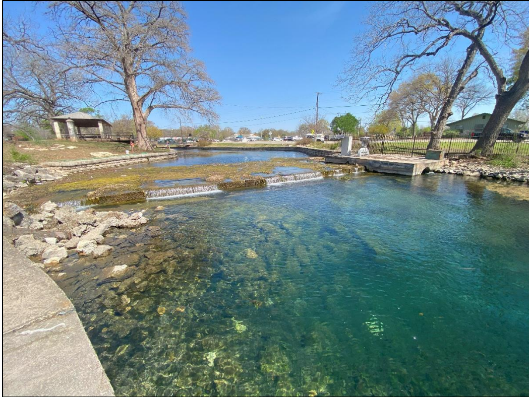
Figure 22. Water flowing over the weir dam in the New Channel at 70 cfs (March 19 th ).
