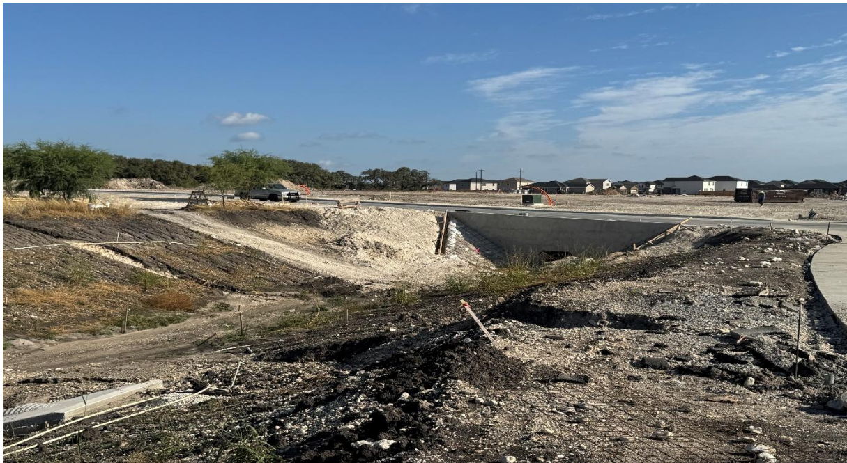
Exhibit C: Installation of Residential Drainage Feature
