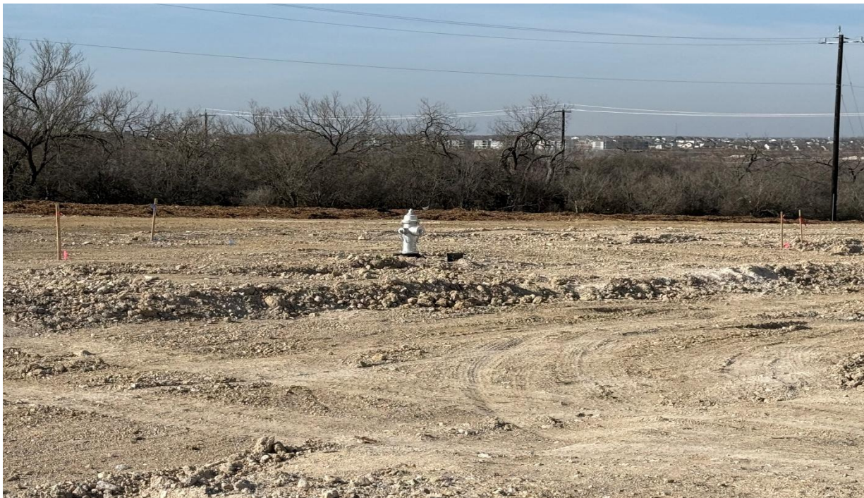
Exhibit E: Water Line Installation and Graded Topsoil
